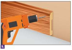
If you wish to use nails, avoid placing them in the backside groove of the profiles.
